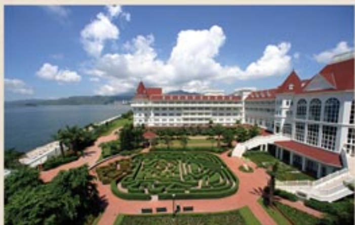
Hong Kong Disneyland Hotel
